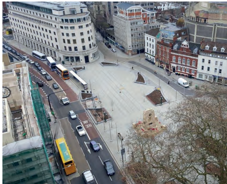
City centre- before layout with the scissors junction ( left ) and after, created simplified, largely segregated routes for buses, pedestrians and cyclists ( right )
